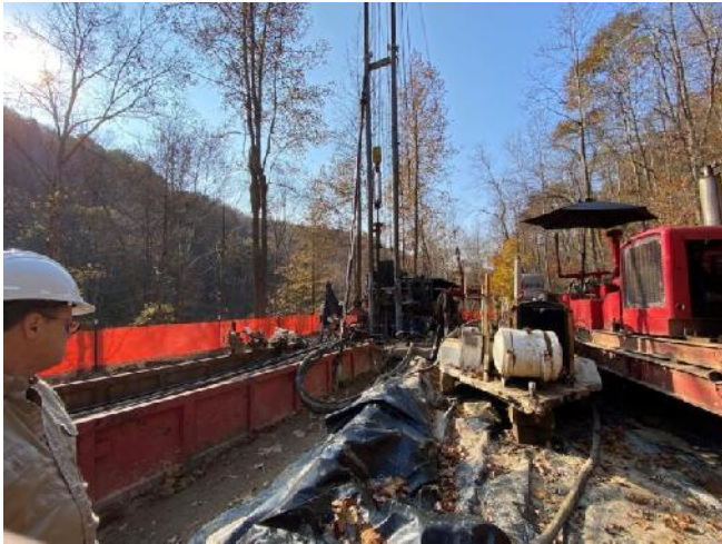
An orphan well plugging operation in Vinton Furnace State Forest in fall 2021. (Auditor of State Keith Faber's Office)
