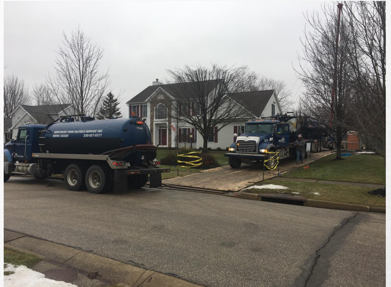
2018 Project: Portage #1 Dunlap #2 (1 of 3) Contractor: GonzOil, Inc. Project Status: Completed
