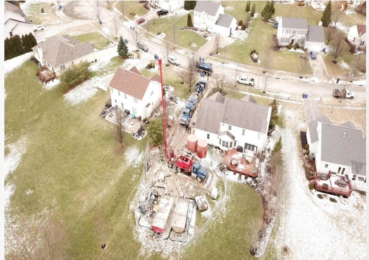
2018 Project: Portage #1 Dunlap #2 (1 of 3) Contractor: GonzOil, Inc. Project Status: Completed
