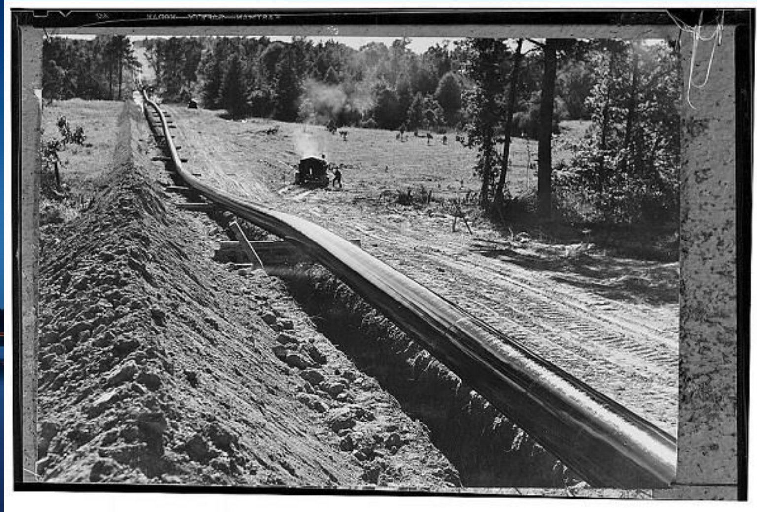
Construction of the First Cross Country Pipeline - During WWII
